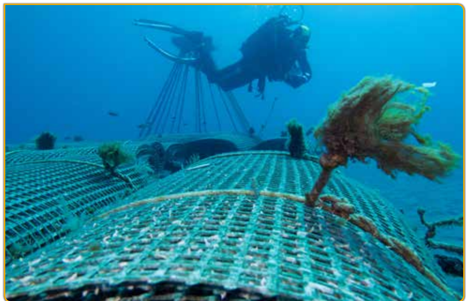
REMORA Project: Consisting of light structures, the reef was designed to provide a habitat and protection to young aquatic life by boosting the fixation of microfauna, microflora and postlarvae, thus providing nutrients to both the fish and the seabed.
